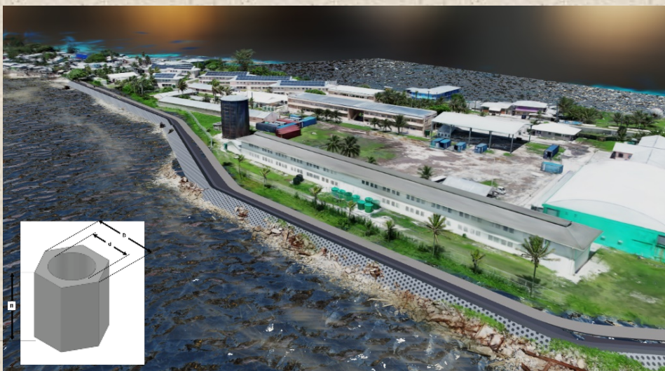
Figure 2 Seabee revetment at Marshall Islands High School, Majuro
